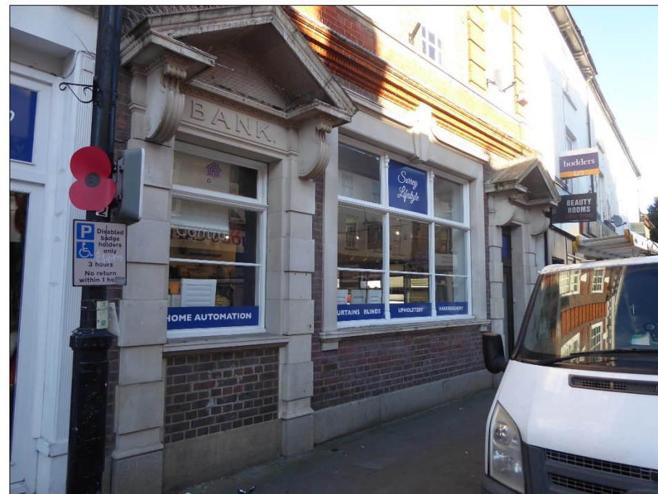
Figure 11: Stone cladding to 125, Guildford Street
